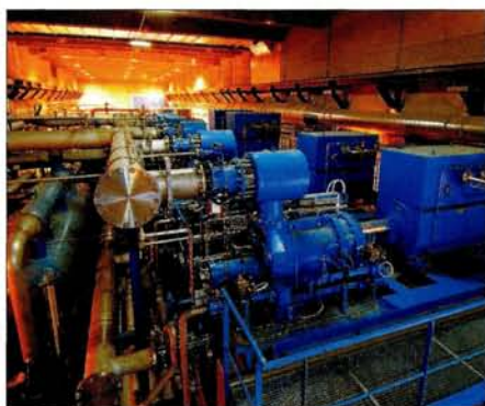
Each of the eight 4.5 K refrigerators for the LHC consists of a compressor station (left) and a cold box (Air Liquide, middle; Linde, right).
