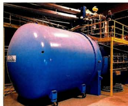
Each of the eight 4.5 K refrigerators for the LHC consists of a compressor station (left) and a cold box (Air Liquide, middle; Linde, right).
